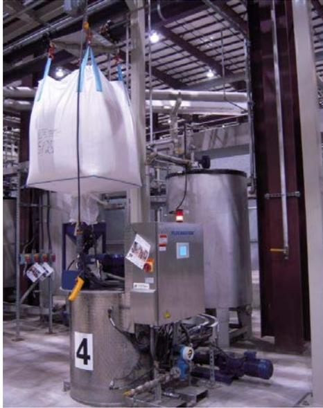
**Figure 3. Flocculant dosing station**
