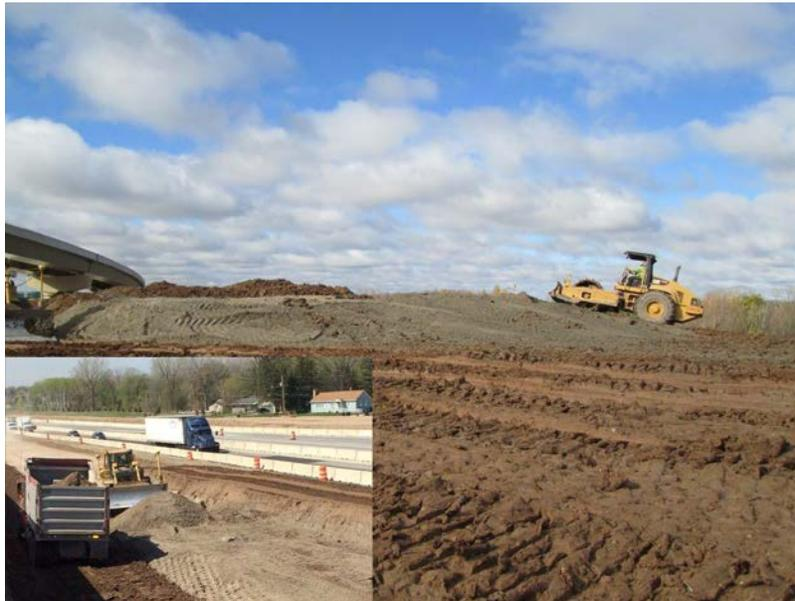
**Figure 5. Approved sand from the Lower Fox River remediation project being incorporated into the road base construction at the approved WisDOT project**
